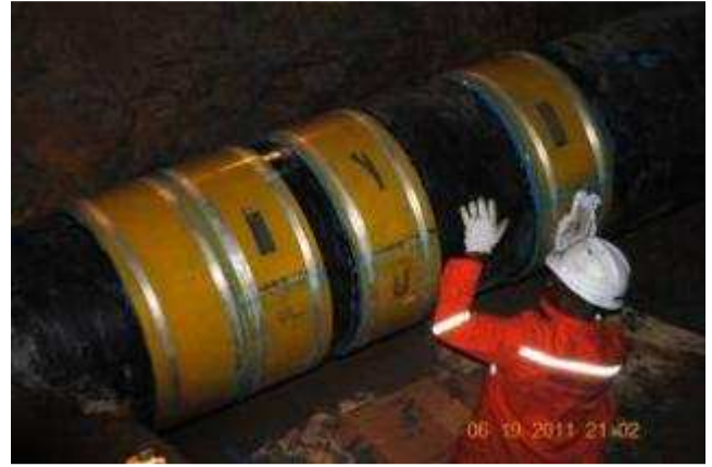
Figure 7. Completed 28" repair sleeve installation
