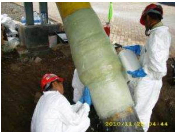
Figure 16. Contour – insulating joint repair
