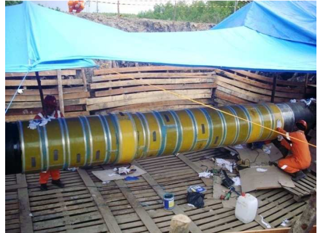
Figure 3. Installation of repair sleeves on the 28" gas line
