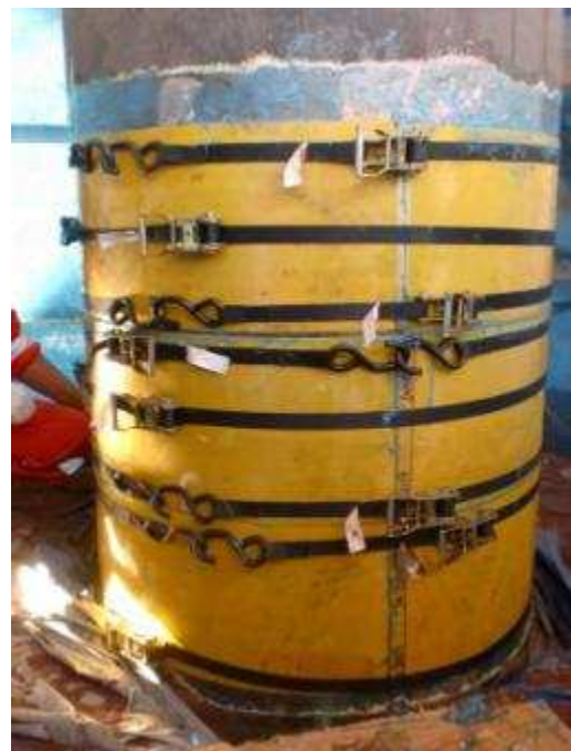
Figure 11. Sample of completed sump caisson repair
