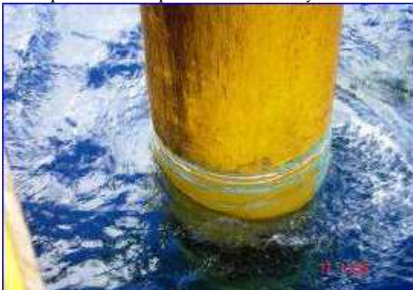
Figure 10. Completed 42" Skim Pile repair
