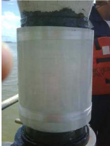
Figure 9. Completed high temperature composite sleeve repair
