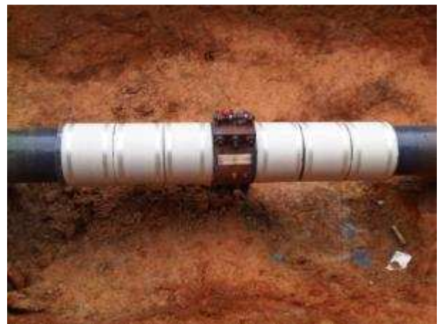
Figure 15. Completed 12" Crack Arrestor repair
