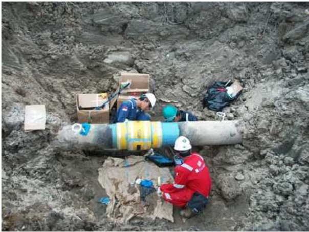
Figure 12. Completed girth weld repair
