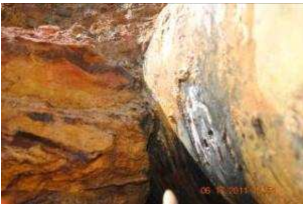
Figure 6. The alkaline soil erosion type defect
