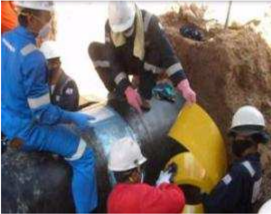
Figure 5. Installation of the 32" seam sleeve
