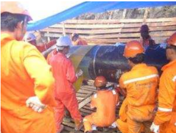
Figure 2. Installation of repair sleeves on the 28" gas line
