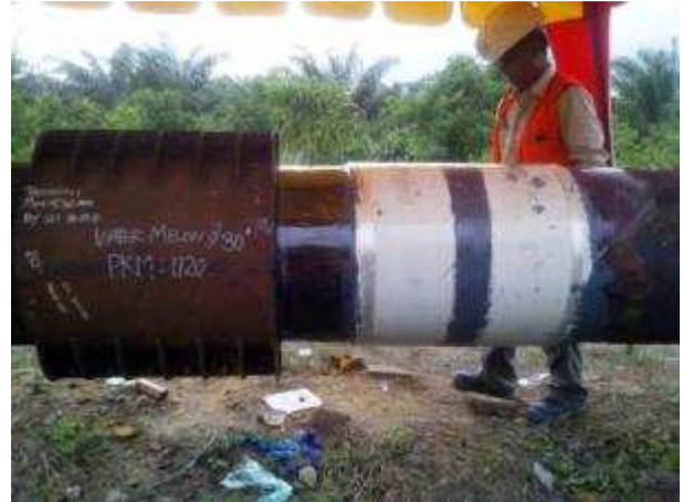
Figure 14. Completed high temp repair
